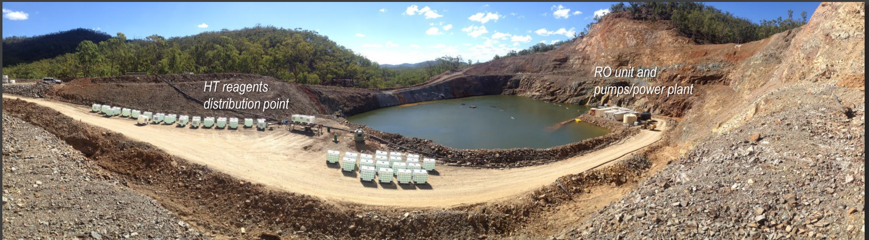
HT technology implementation at commencement
