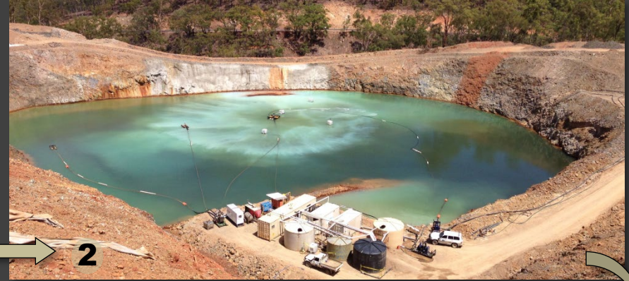
Pit during treatment with white halo highlighting hydrotalcite precipitating in-situ.
